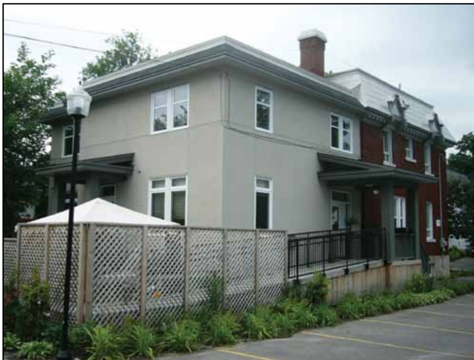
Transition House as it is today, featuring the expansion
